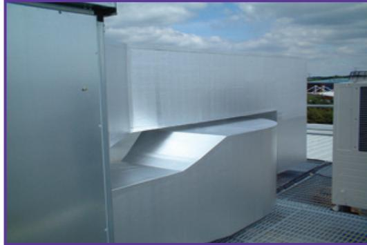
VentureClad® 1577CW is a zero permeability, absolute vapor barrier for insulation cladding and jacketing applications. A 5-ply, self adhesive material installs quickly and easily with no special tools required, resulting in significant time, labor, and cost savings.
